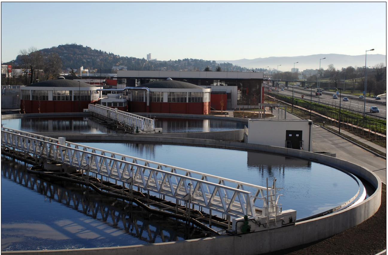
Station d'épuration Furania
